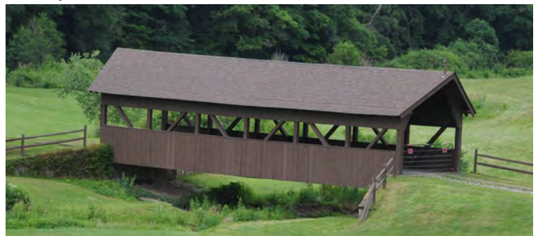
Hoffarosa covered bridge
